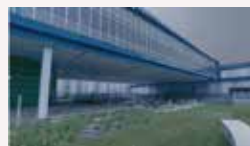
TERRESTRIAL LASER SCANNING
